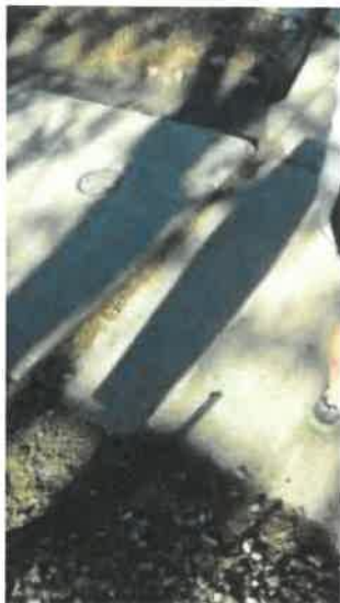
Figure 4a 2088 Niagara Falls Blvd
