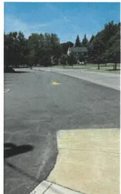
Figure 7a South side of Irvington Drive
